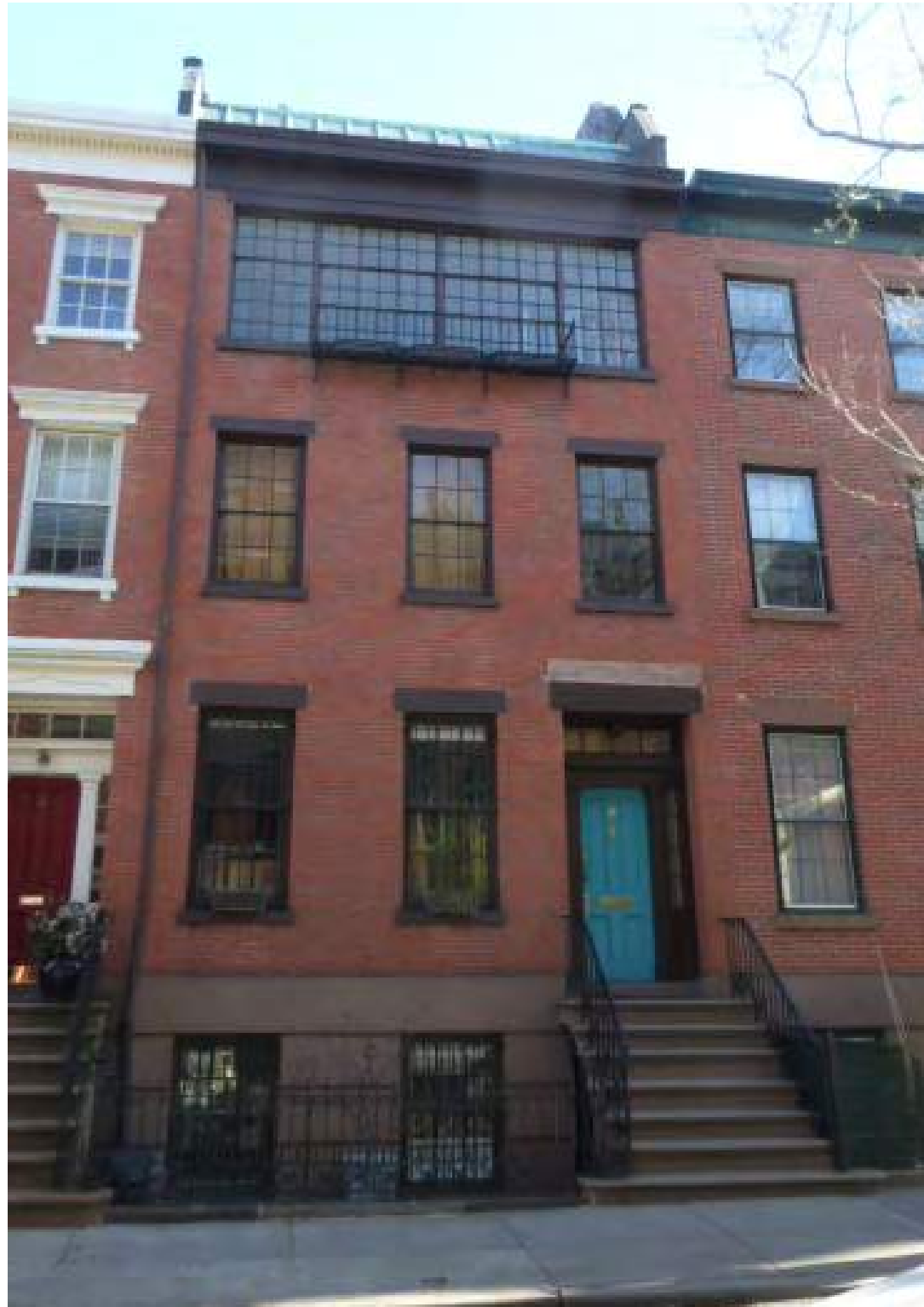
34 Perry Street - Studio window added C.1924
