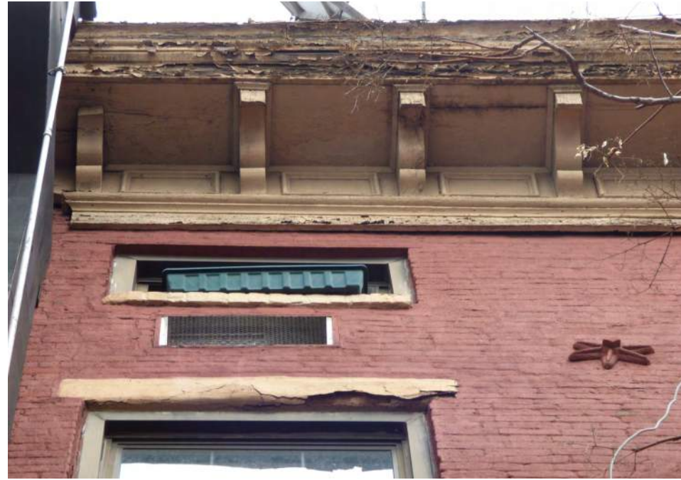
Existing condition - deteriorated wood cornice and deteriorated brownstone lintels
