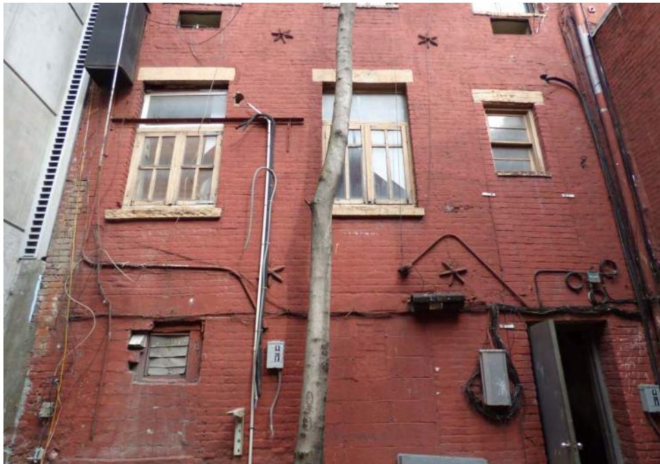
Existing overall view of cellar and first floors
