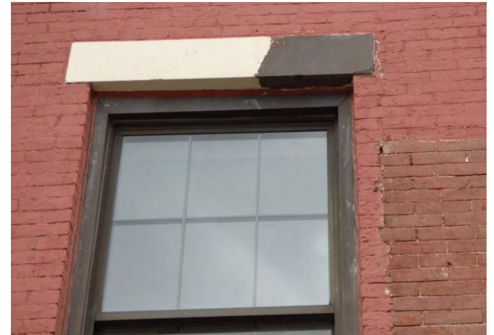
Probes at existing façade revealed non-historic lintels and original brick behind paint coatings
