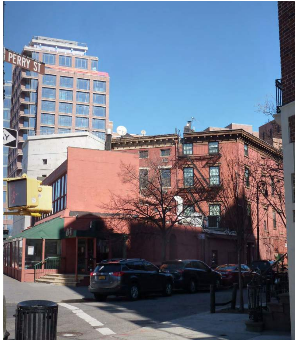
Existing Rear Façade
