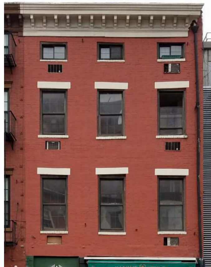
Existing overall view of second to fourth floors
