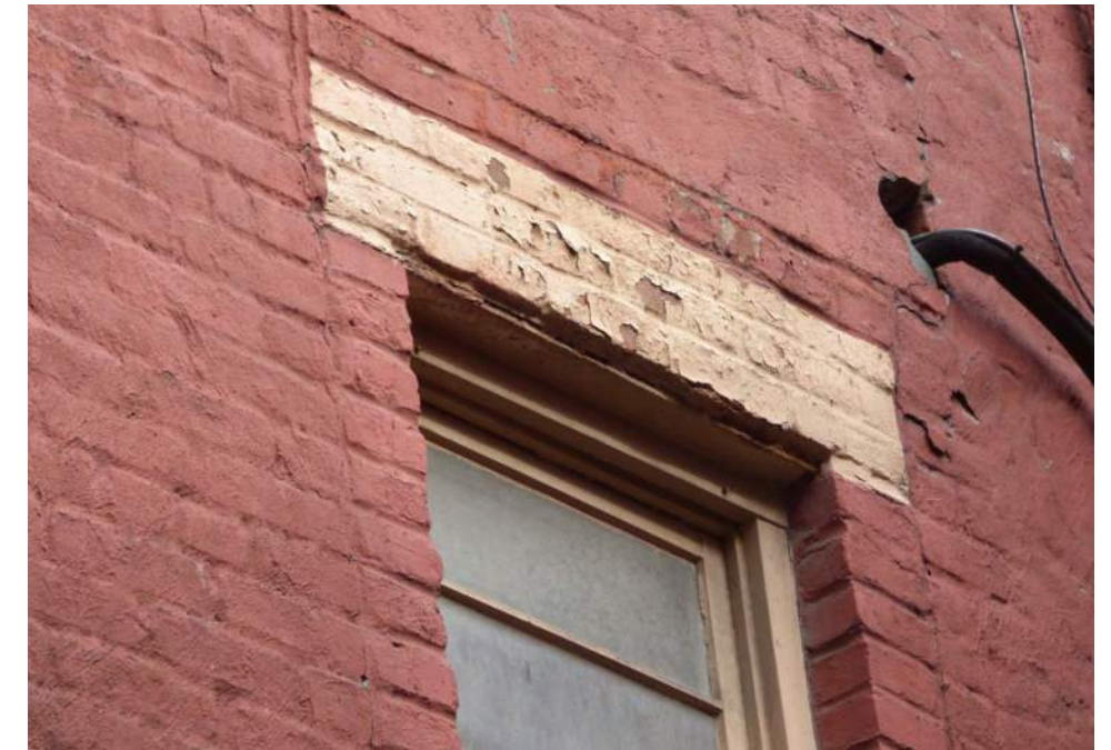
Existing condition - partially infilled masonry opening
