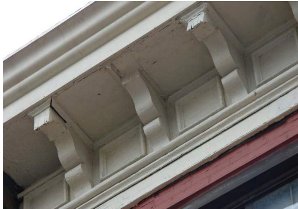
Existing cornice condition - missing wood elements
