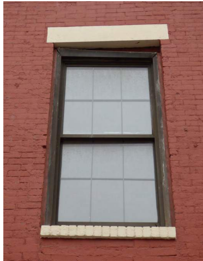
Existing window condition - metal windows, brick sills, replaced lintels
