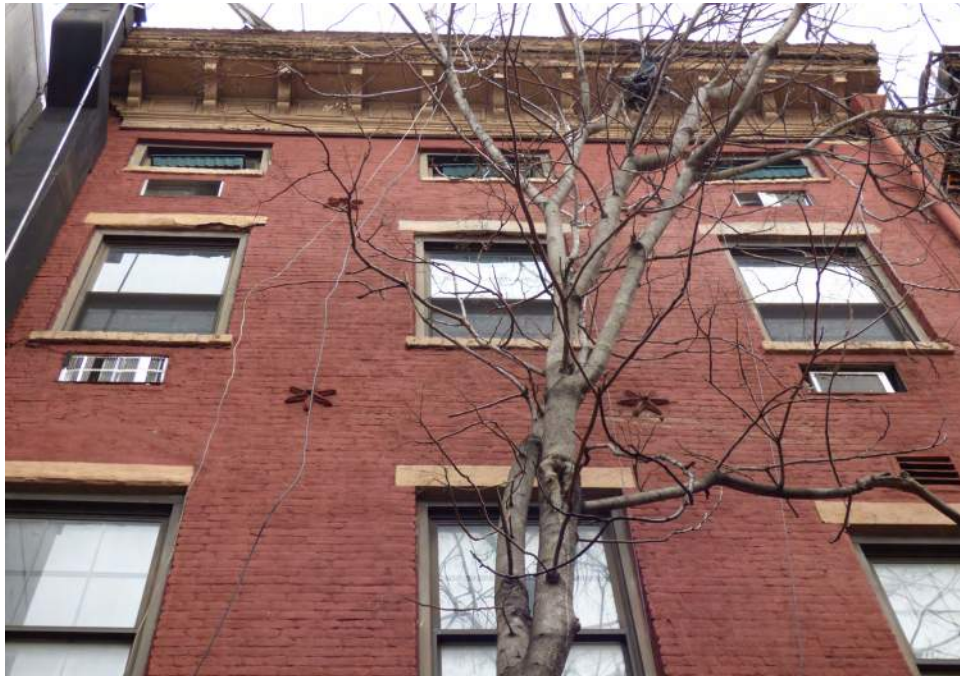
Existing overall view of second to fourth floors
