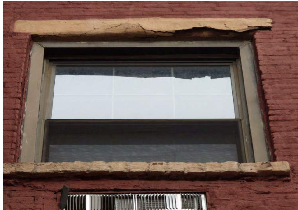
Existing window condition - metal windows, brick sills, deteriorated brownstone lintels
