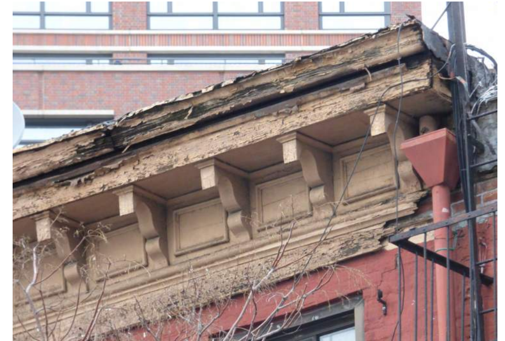
Existing cornice condition - deteriorated wood elements
