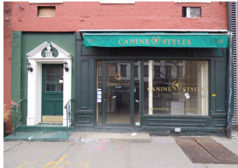
Existing first floor/storefront condition
