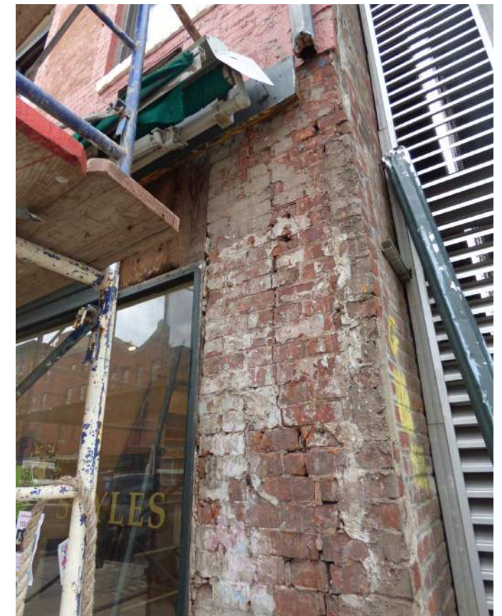
Probe at existing storefront revealed deteriorated brick piers
